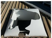
The first incident occurred when a contractor fell backwards through an unprotected skylight, falling 4.6m and sustaining multiple fractures. The contractor was inspecting anchor points on the roof at the time.
